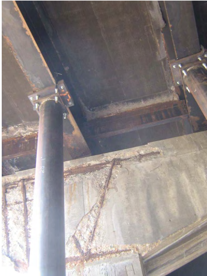
5. Underside of Bridge on the South Side
