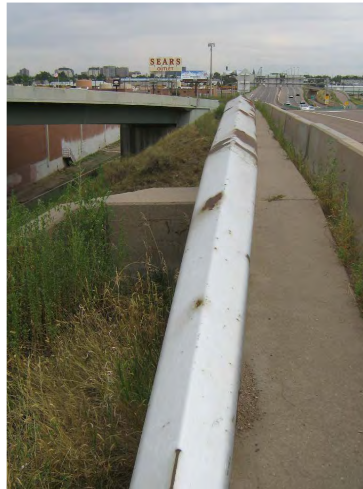
2. Pedestrian Walkway on the North Side of Bridge
