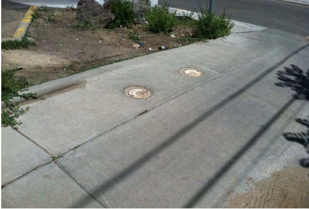
Photo 1 (438 Federal Boulevard) – View of monitoring wells located in alley behind Conoco gas station
