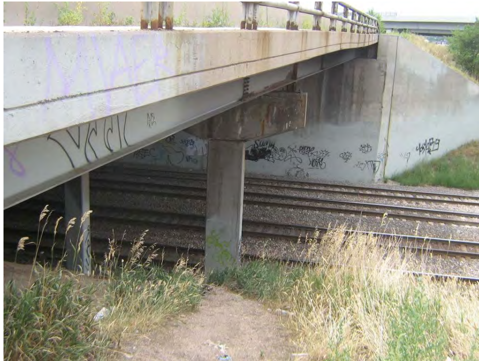
3. Looking at the West Side of Bridge
