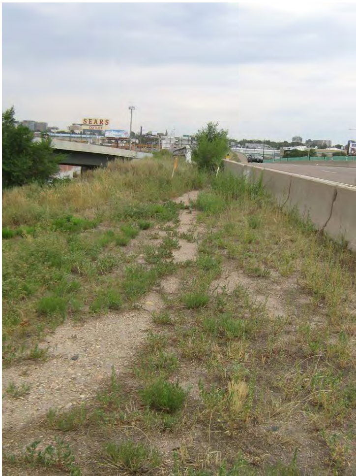
1. North Side of Bridge, Looking East
