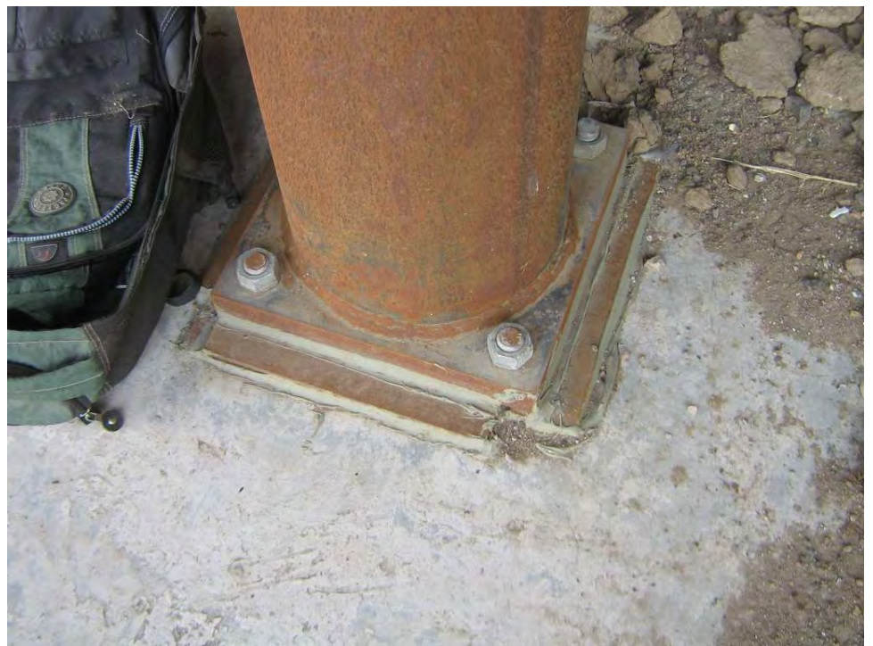
6. Caulking on Bridge Pier at the South End
